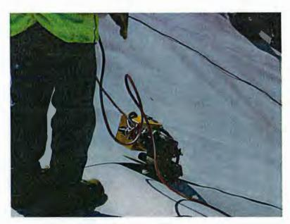
Thermal fusion welding apparatus
