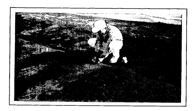
Figure 6.11 - Photograph of Geonet Joining by Using Plastic Fasteners
