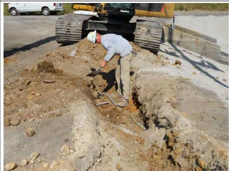
Abandoned 8 inch diameter pipe near the North Concrete Inlet Structure, looking south
