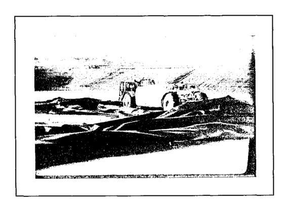
Figure 3.18 - Wind Damage to Deployed Geomembrane
