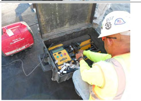
Performing non-destructive air testing of the geomembrane fusion welded seams
