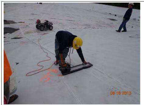
Installing geomembrane pipe boot around marker post, looking east
