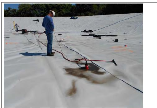
Extrusion welding geomembrane repair, looking east
