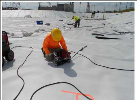
Nondestructive testing geomembrane fusion welded seam, looking southeast
