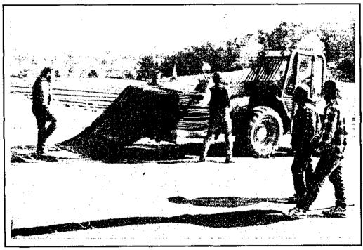
Figure 3.16 - Photographs Showing the Unrolling (Upper) and Unfolding (Lower) of Geomembranes
