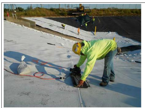
Geomembrane trial weld prior to production seaming, looking southwest
