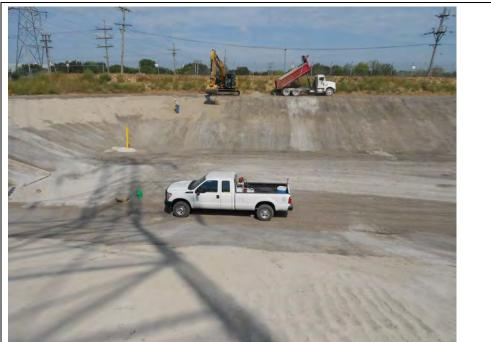
Moisture conditioning screenings placed in sump prior to compaction, looking northwest
