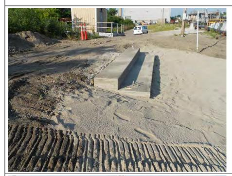
Preparing concrete surfaces for geomembrane batten connection, looking southwest
