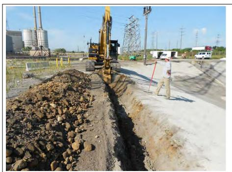
Hand exposing damaged utility south of the North Concrete Inlet Structure
