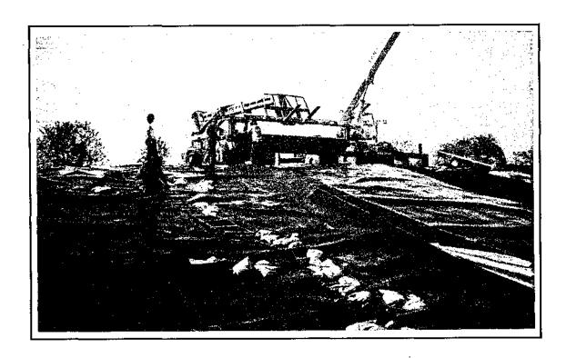
Figure 3.17 - HDPE Geomembrane Showing Sun Induced Wrinkles
